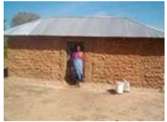
This is Kanze Mramba outside her new house which she managed to construct after taking loans from Lamukani SHG and engaged herself into business ventures which enabled her purchase iron sheets for this house.
